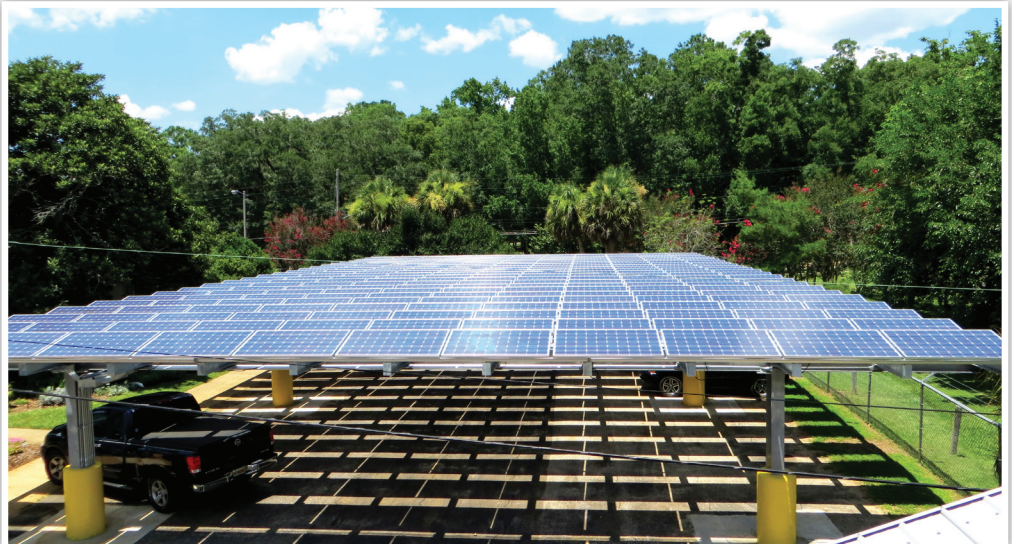
Leon County Cooperative Extension Net-Zero Facility
